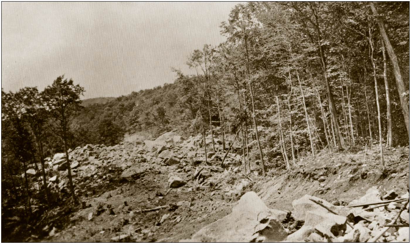
To build the new Route 10, workmen blasted through Green Mountain in 1941.
