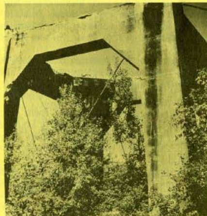
Remains of Surge Tower near Sprite Creek
