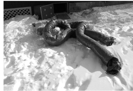
Old Flex Ducts
